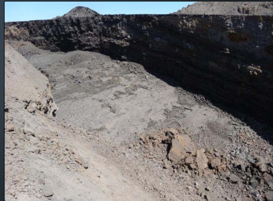
Close-up of bedding shear (dip \pm 15^\circ flattening to \pm 8^\circ towards failure toe)
