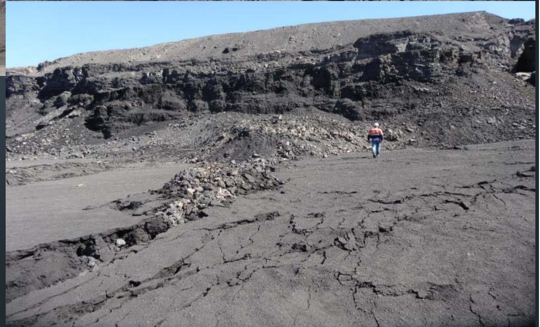
Compression features along top edge of failure
