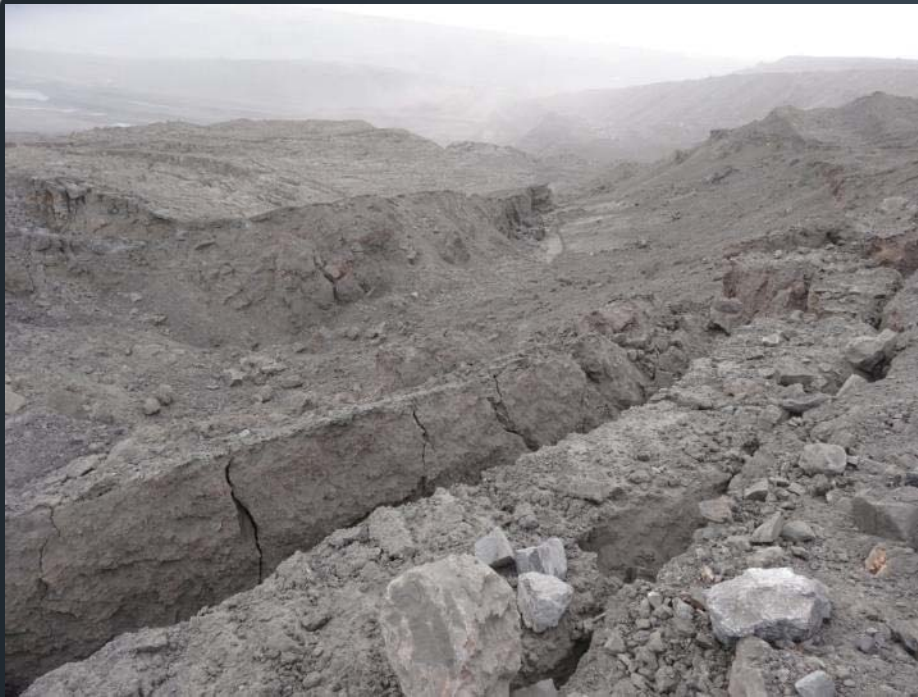
Top of boxcut ramp failure
