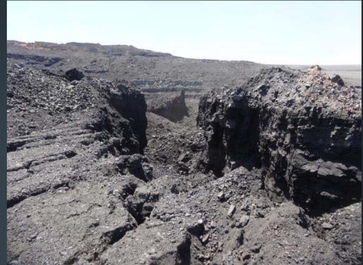
Crack through ramp at base of failure
